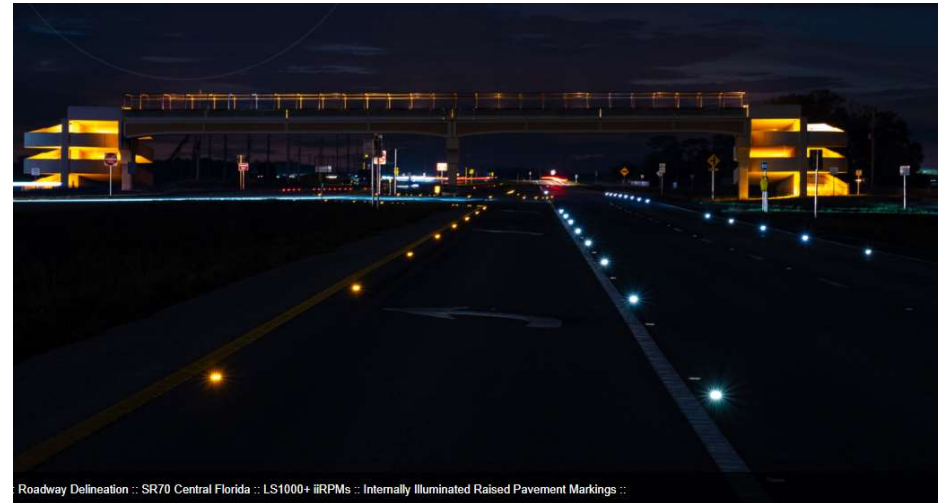
Roadway Delineation :: SR70 Central Florida :: LS1000+ iIRPMs :: Internally Illuminated Raised Pavement Markings ::
